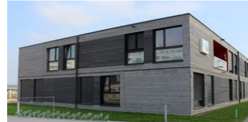
PopUp dorms: Flexible wooden pre-fabricated container constructions (2015)
